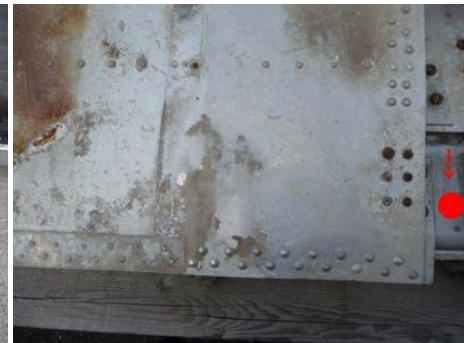
Lower wing boxes - work to do
